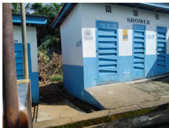
Figure 15: Ramp built in Goderich but still not accessible for a wheelchair user.
